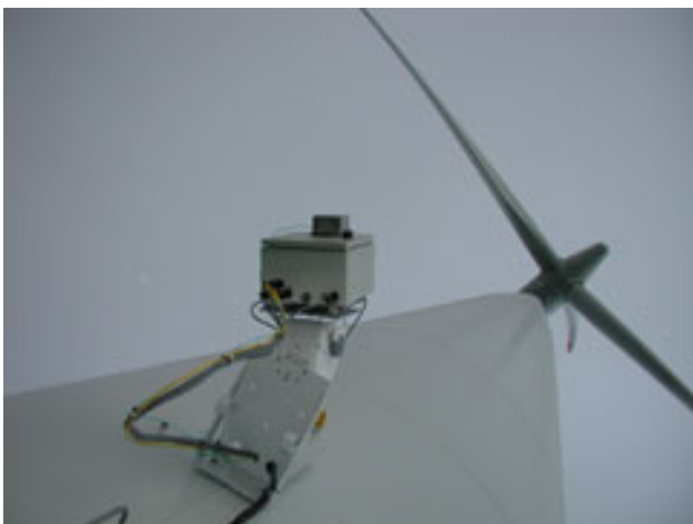
Figure 3. Thermal camera mounted with a pan/tilt head on an offshore turbine at Nysted wind farm.
